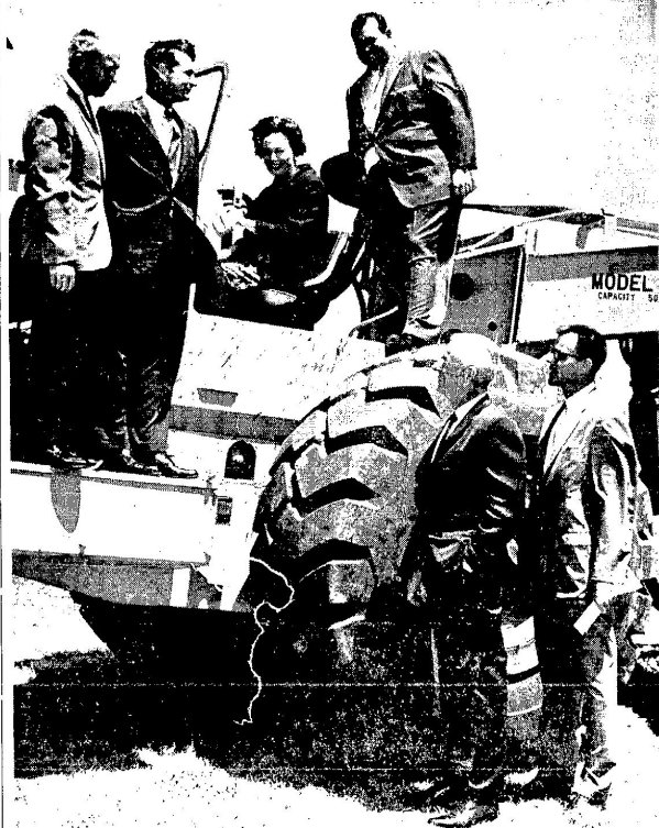
VOCATIONAL CENTER... At the throttle as ground is broken for Hayward Unified School District's vocational skills center is HUSD Trustee Suzanne Clemens. Also participating in yesterday's ceremonies at the site, 26316 Hesperian Blvd., Hayward, are, from left, Ami Pelton of Hayward Chamber of Commerce; HUSD Trustee Ray Baker; Hayward Vice Mayor Jack Smith; Robert S. Ash, executive secretary of Alameda County Central Labor Council, AFL-CIO, and HUSD Dist. Supt. Dr. William Cunningham. —Review Photo
