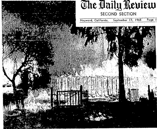
RUSSELL CITY AGAIN . . . The largely deserted Russell City area west of Hayward, where little remains to burn, was the scene of another wild blaze last night. Alameda County Fire Patrol estimated that another dozen abandoned buildings were destroyed.
