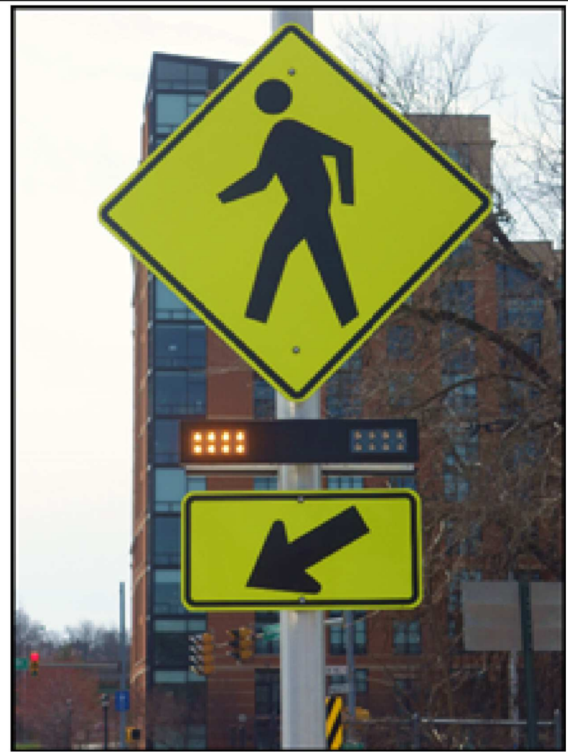
Rectangular Rapid Flashing Beacon (Long-Term)
