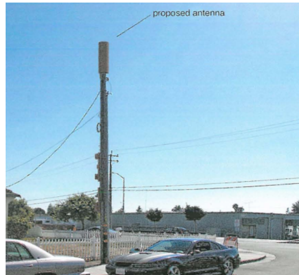
EXAMPLE: Top Mounted Antenna
