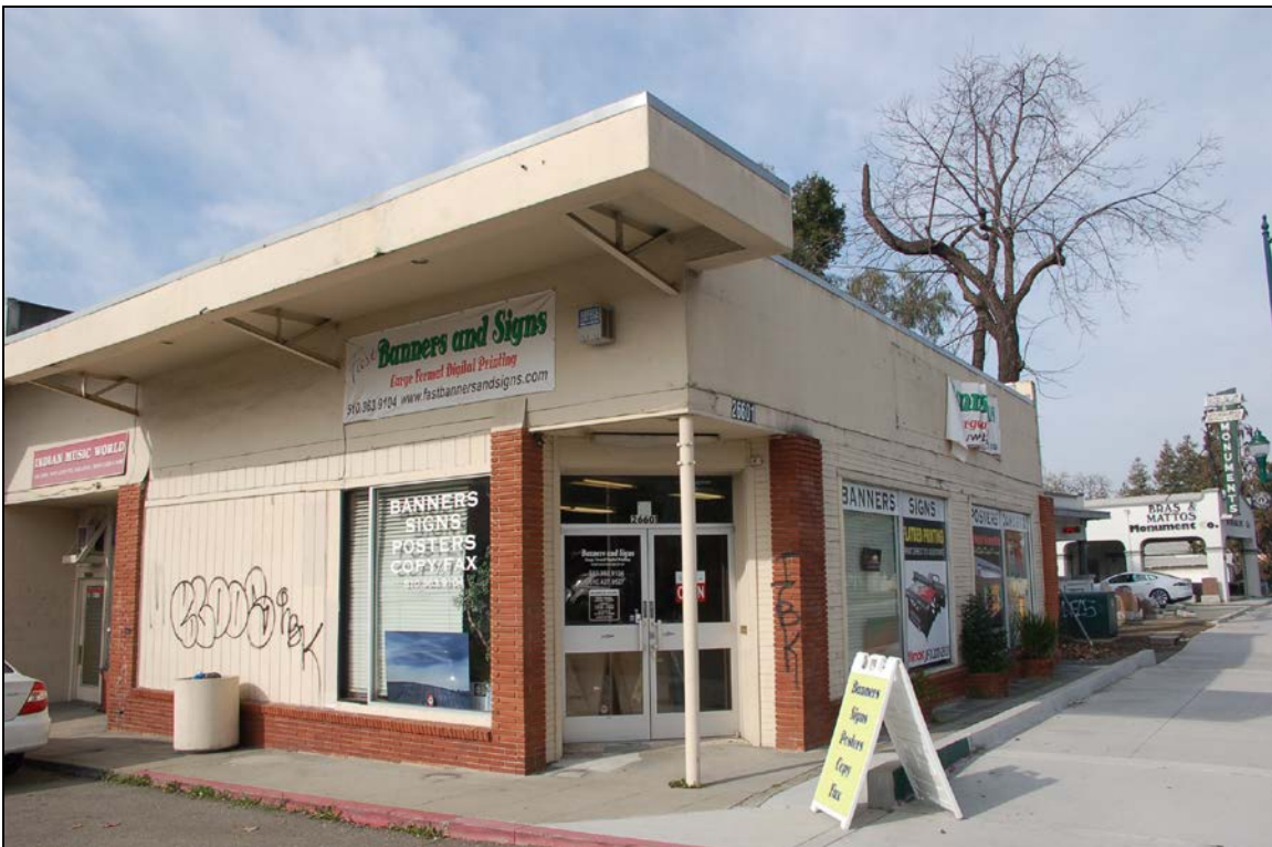
26601 Mission Blvd, north end of building – view to the northwest
