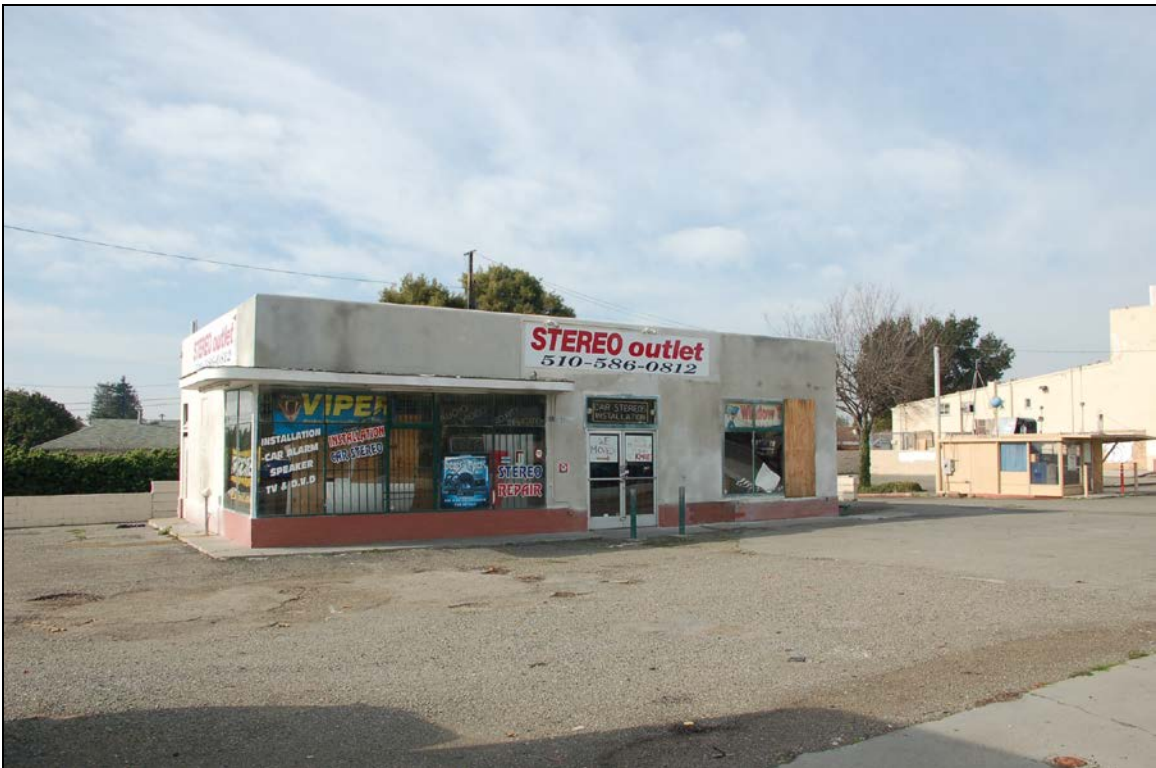
Figure 9: 26699 Mission Blvd, former Texaco gas station – view to the west
