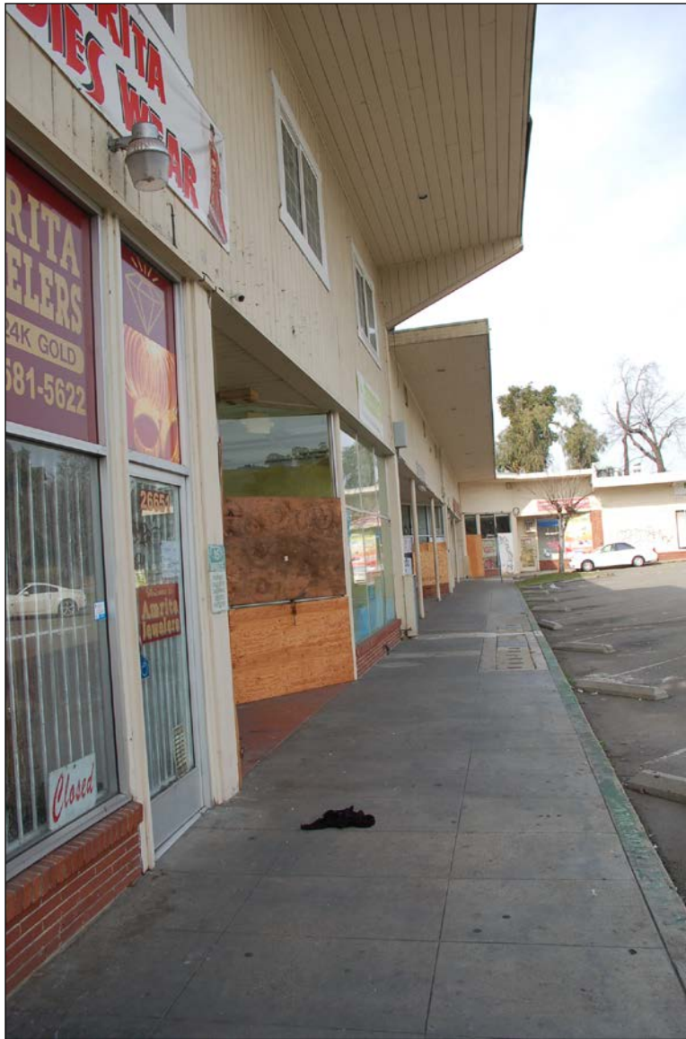
26601-26671 Mission Boulevard, view north along building façade
