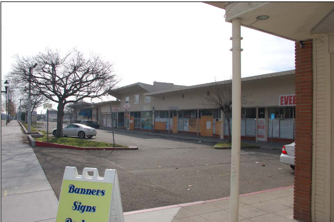
Figure 5: 26601-26671 Mission Blvd, view to south of shopping center from north end
