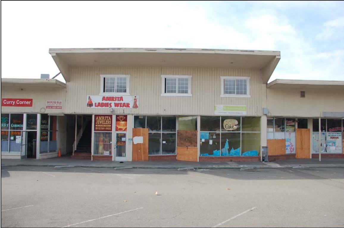
Figure 6: 26601-26671 Mission Blvd, two story section – view to west
