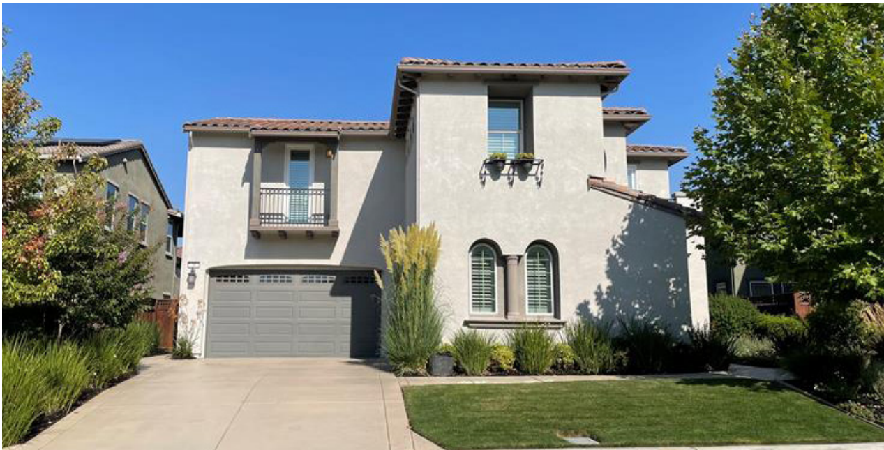
Example of of a single family home with the garage setback further from the primary building.
