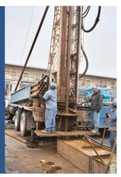
Drilling operation for nested monitoring well
