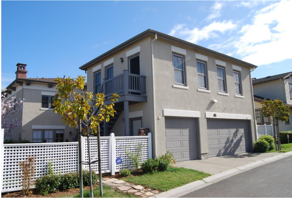
Two-story Carriage Building with living unit above
