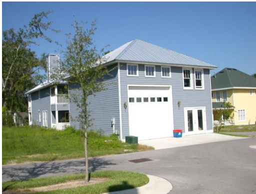
Two-story Carriage Building with living unit above
