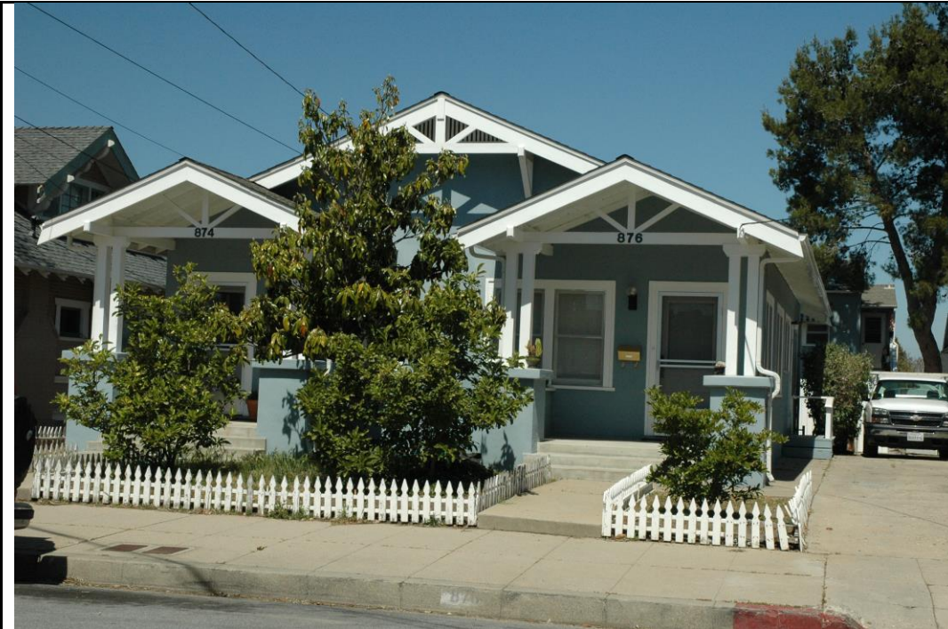
Duplex side-by-side units, each with projecting porch.
