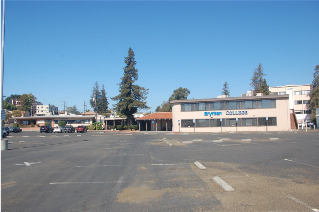
Photo 3: 22336 Main Street -view from northeast
