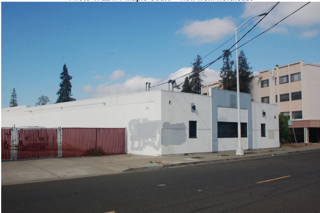
Photo 2: 22477 Maple Court – view from southeast
