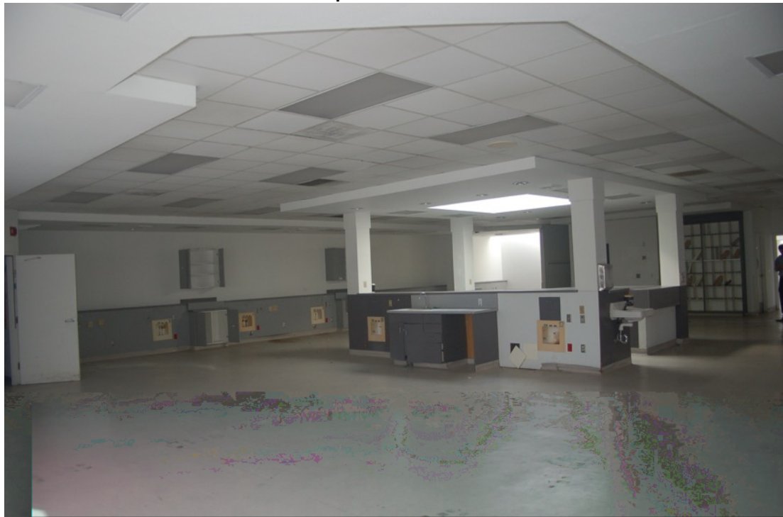
Photo 4: 22477 Maple Court – view from southeast
