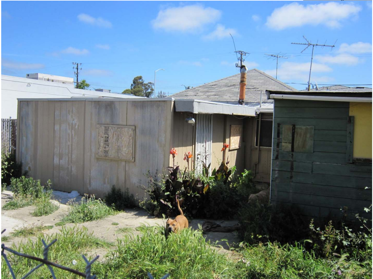
Photograph 6 Property: 22941 Maple Court, Hayward CA View: Rear of the property showing two of the buildings on the site ,both appear to be residential units. Date: April 2015
