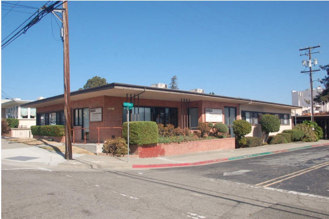
Photo 1: 22330 Main Street - view from southwest
