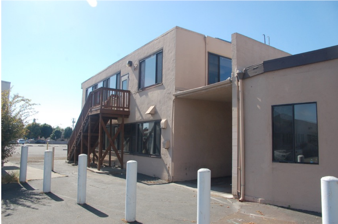
Photo 5: 22336 Main Street – view from northeast
