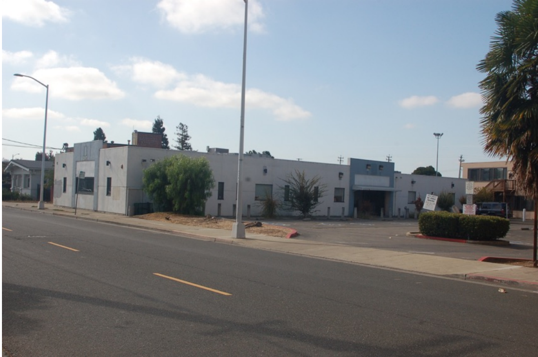
Photo 1: 22477 Maple Court – view from northeast
