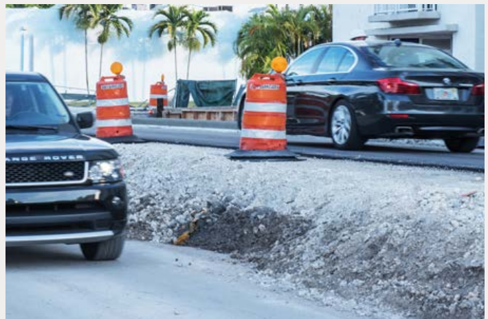
Raised road during construction ( http://www.mbrisingabove.com/ )
