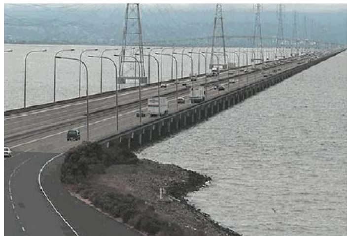
State Route 92 bridge approach heading toward San Mateo (CA COT, 2019)
