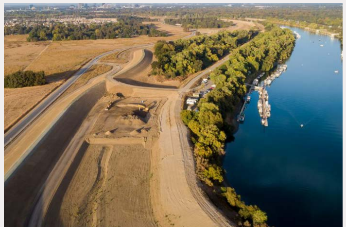
Sacramento River levee
