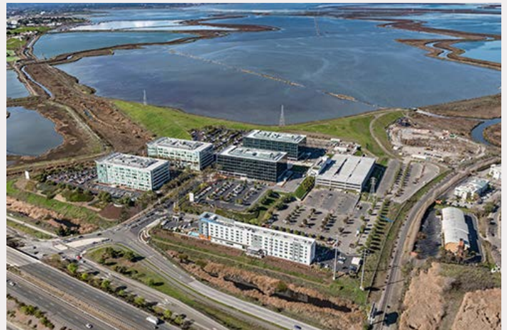
Access roads were raised to reach the higher elevation ( www.steelwavellc.com )
