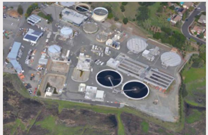
Aerial view of upgraded plant (Novato Sanitary District)
