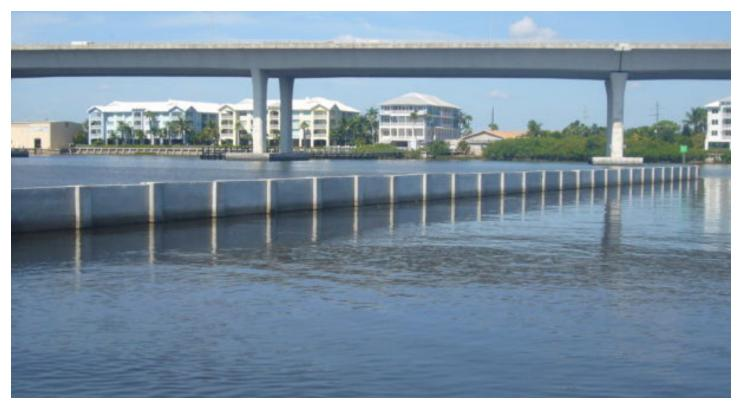
Wave screen along the perimeter of the basin, made of all concrete
