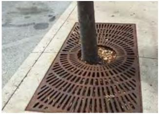
Example tree well filtration (https://nacto.org/publication/urban-streetstormwater-guide/stormwater-elements/green-stormwater-elements/ stormwater-tree/, right: http://www.ironsmith.cc/TREE-GRATES-STARB.htm)
