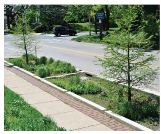
Bioretention bulbout in Philadelphia, PA (https://nacto.org/publication/urban-street-stormwater-guide/stormwater-elements/green-infrastructure-configurations/stormwater-curb-extension/)
