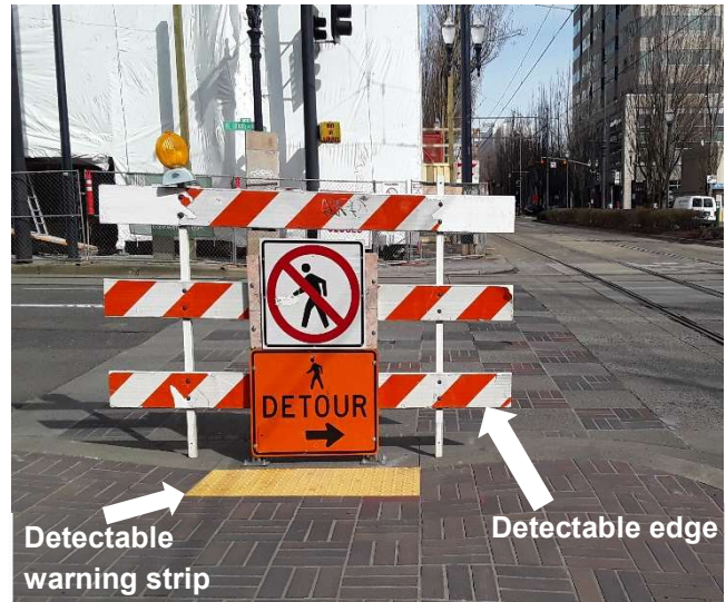
Figure 11. A barricade with a detectable edge and a curb ramp with detectable warning strip.
