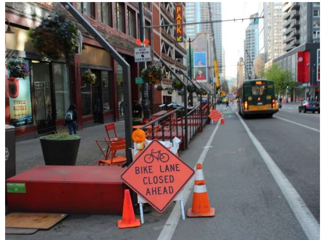
Figure 23. Signs should not be placed in a manner that obstructs a pedestrian or bicyclist's travel path. Note that the sign shown is a modified C20 sign and is not CA-MUTD compliant.
