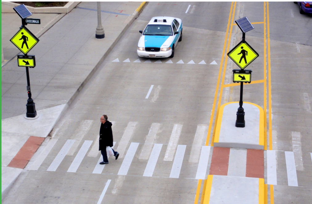
RRFB Device and Markings.
