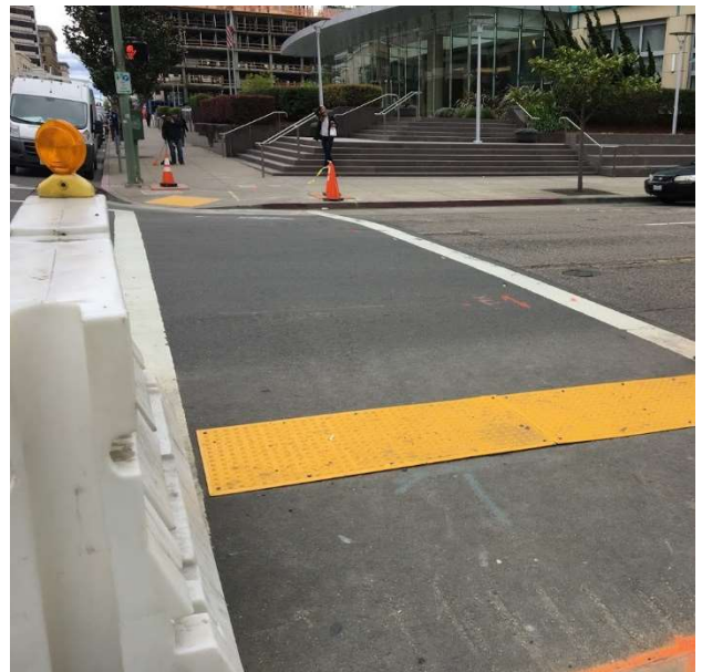
Figure 1. Detectable warning strip clearly marking the start of the exposed crossing to pedestrians with vision disabilities.
