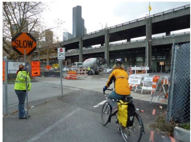
Figure 24. A flagger is used to help bicyclists navigate a difficult intersection which crosses a popular bicycle path.
