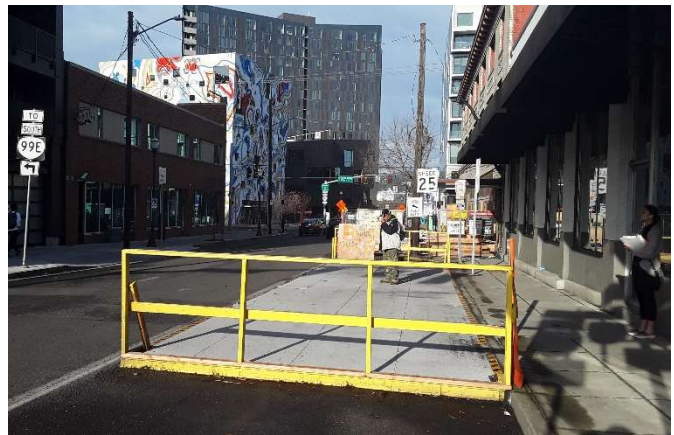
Figure 10. Example of a temporary transit platform created to maintain transit access while the sidewalk and roadway immediately in front of the transit stop are temporarily closed.
