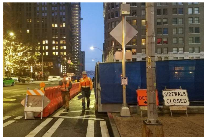
Figure 6. Example of a loading zone used as pedestrian detour while a sidewalk is temporarily closed.
