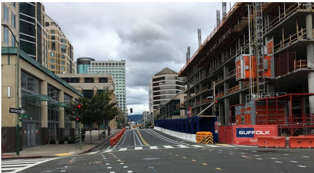
Figure 15. A parking lane is temporarily repurposed as a pedestrian pathway so that the existing bike lane can remain in place despite the adjacent work zone.
