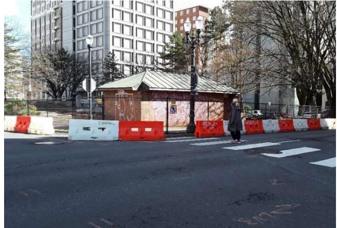
Figure 9. Crashworthy channelization devices are appropriately used to delineate a safe pedestrian pathway but leave room for pedestrians to access the existing crosswalks.
