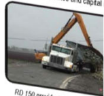
RD 150 provides emergency repairs to levees and drainage infrastructure.
