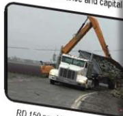
RD 150 provides emergency repairs to levees during flood events.
