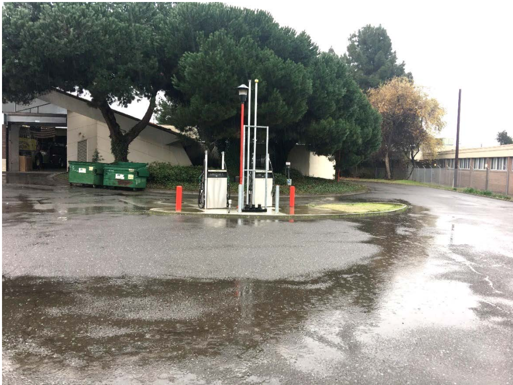
The northwest corner of Fire Station #6 looking south. The street entrance to the Training Facility is on the right. The fuel dispensers and vent pipes for the underground storage tanks are seen in the center. The southeast corner of the Hayward Executive Airport property, adjacent property to the west, is seen in the far right.
