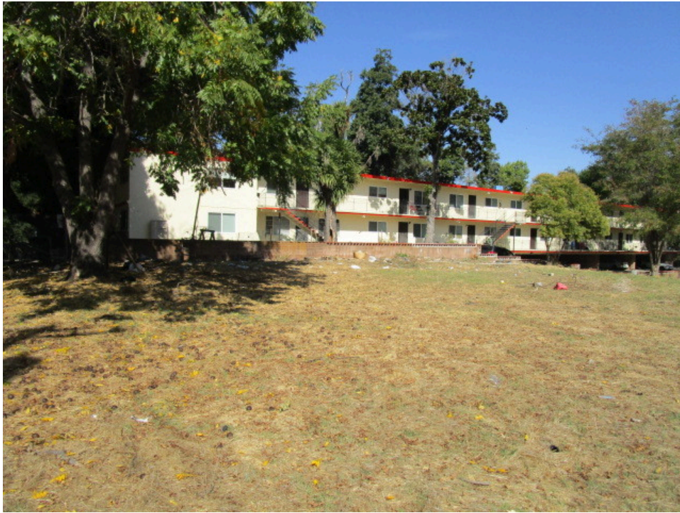
23. The subject property from its southwestern property line (2 of 5)
