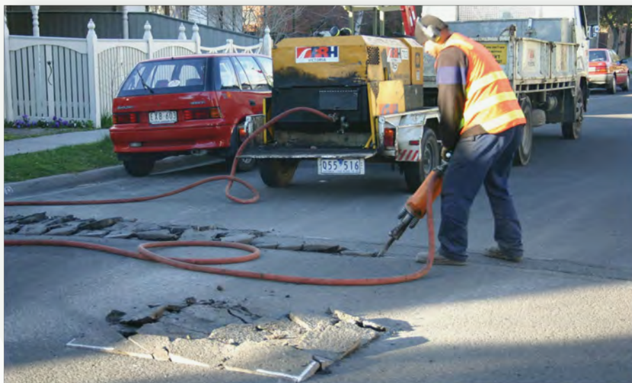
Construction in Hayward
