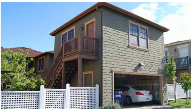
Two-story Carriage Building with small living unit above
