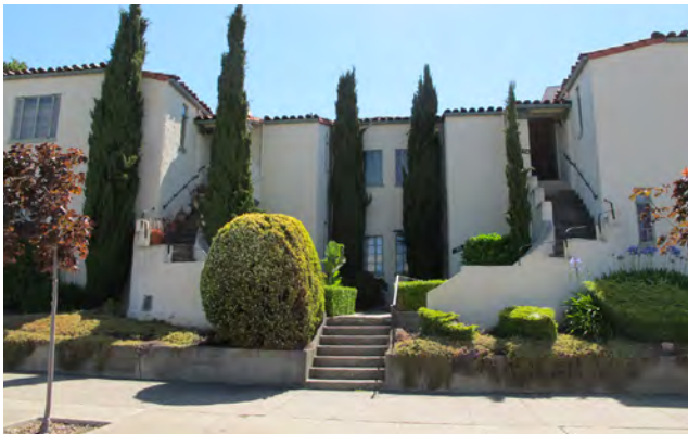
2-story Courtyard building.
