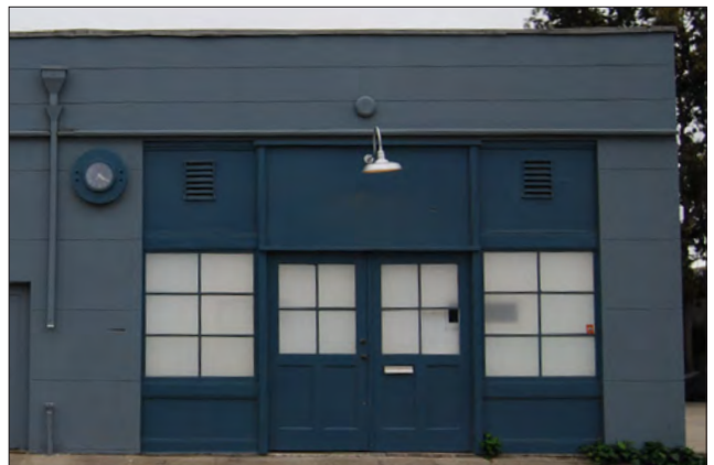
Maker Shopfront with double doors for each entry.
