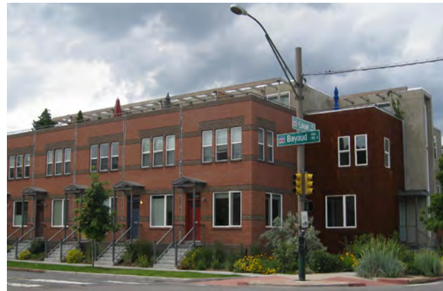
Stoops define the entries to this Rowhouse building while elevating the ground floor from the street level.
