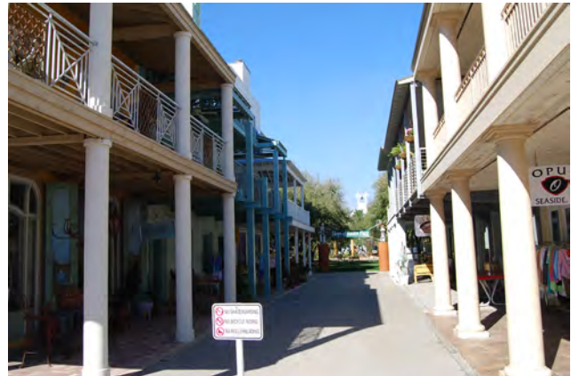
A two-story gallery fronting a passage.
