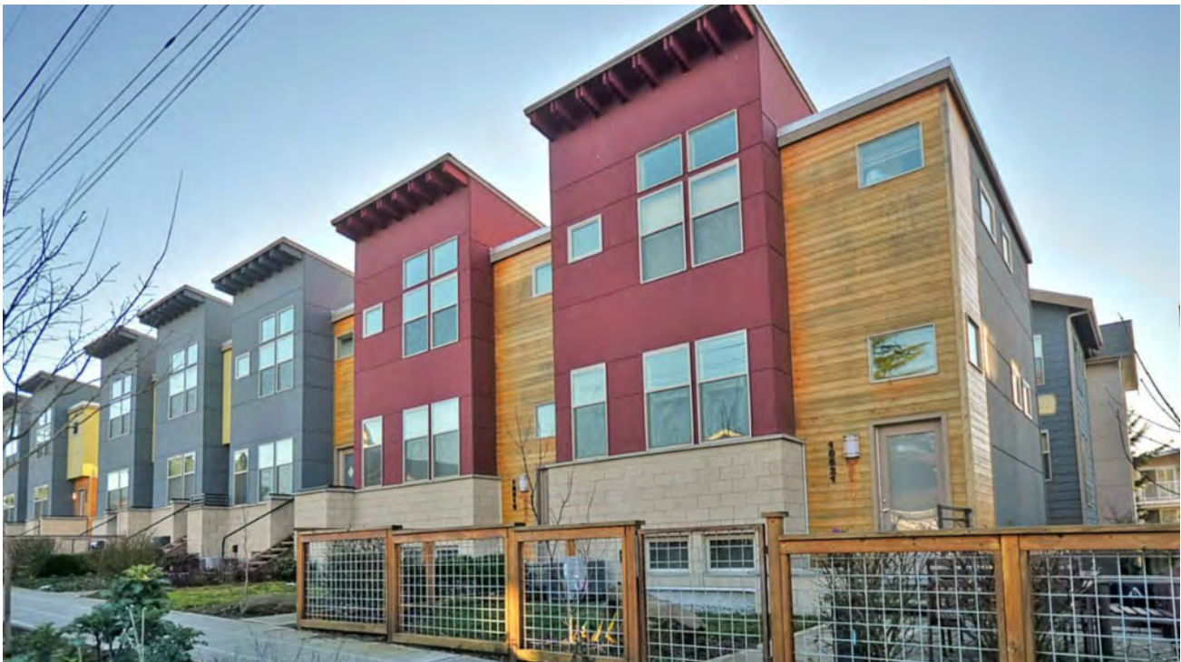
Two-story Rowhouses with stoops that nicely shape this sidewalk.
