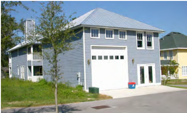
Two-story Carriage Building with living unit above
