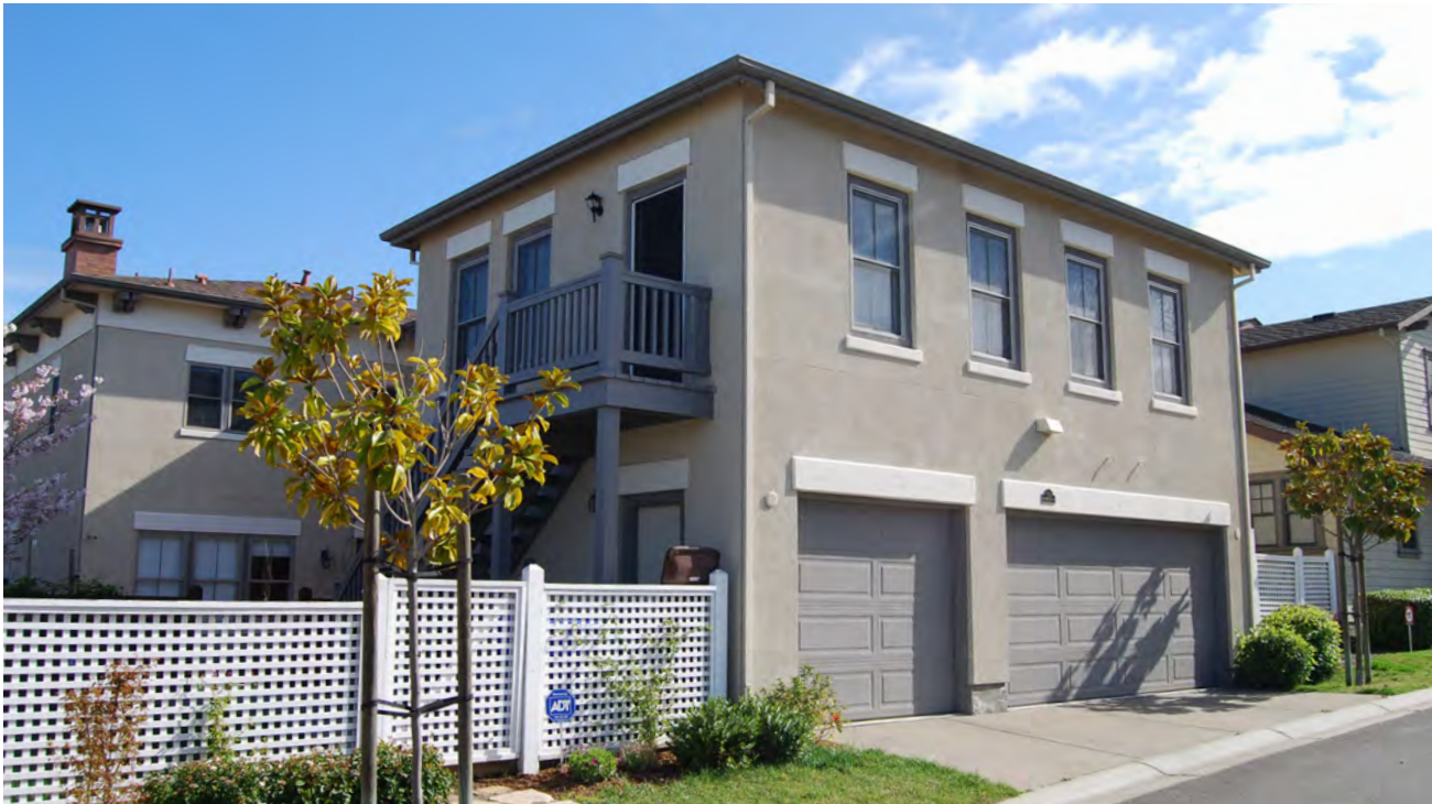
Two-story Carriage Building with living unit above
